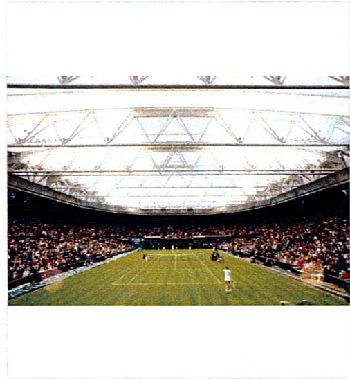
Steffi Graf and Kim Clijsters compete under the new fabric roof at Wimbledon's Centre Court. W.L. Gore Product Specialist Thomas Kelmartin, who works in the company's Appleton South site in Elkton, led the project that created the fabric. PHOTO COURTESY OF W.L. GORE
